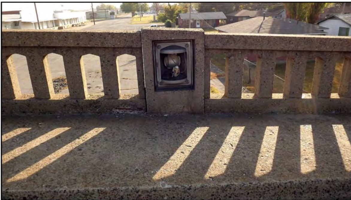
Figure 15. Bridge 2001 Recessed Lighting Unit Roadway Elevation – South End View to the East
