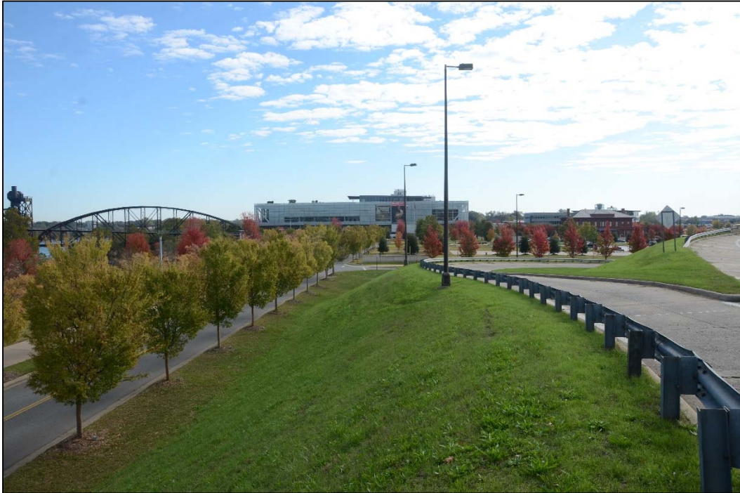
Figure 7: Above-Grade, On-Fill
