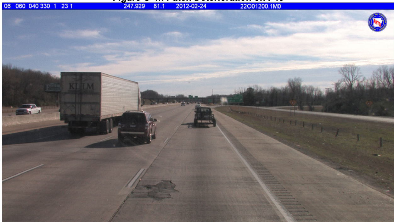
Figure C-4f. Patch Deterioration on I-40
