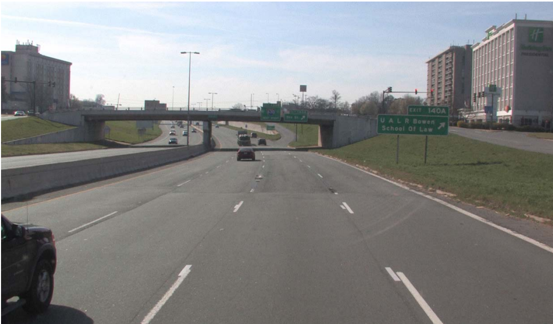
Figure C-5c. Inadequate Shoulders and Curb and Gutter Adjacent to I-30
