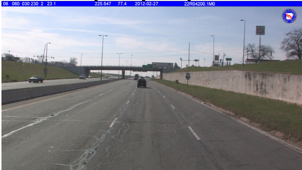
Figure C-4b. Joint Reflection Cracking on I-30
