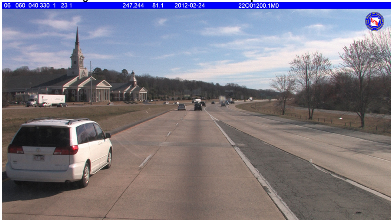
Figure C-4e. Lane and Shoulder Joint Separation on I-40
