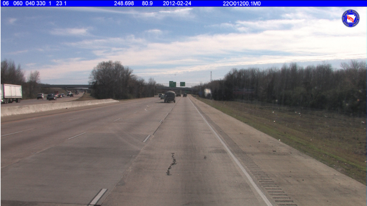
Figure C-4g. Linear Cracking on I-40
