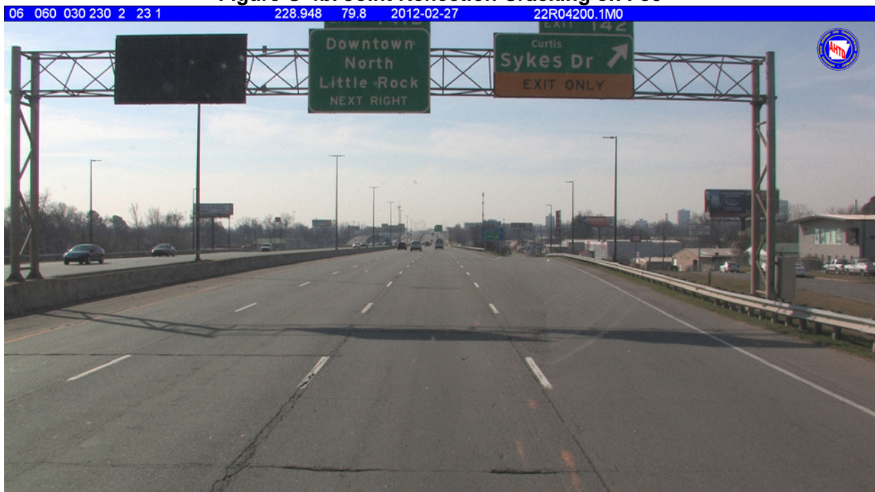
Figure C-4b. Joint Reflection Cracking on I-30
